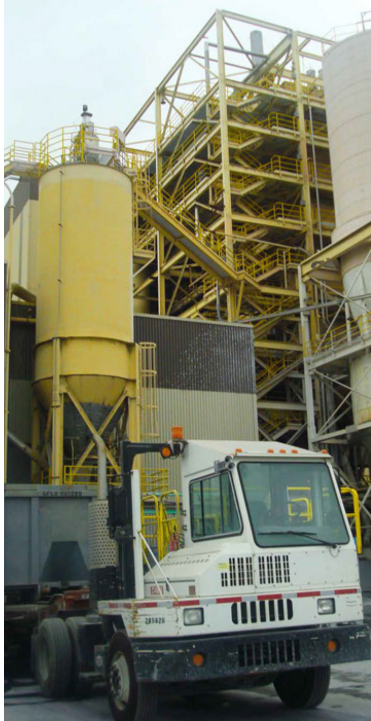
Commerce Refuse-To-Energy Facility (CREF)
