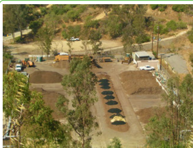
Griffith Park Composting Facility
