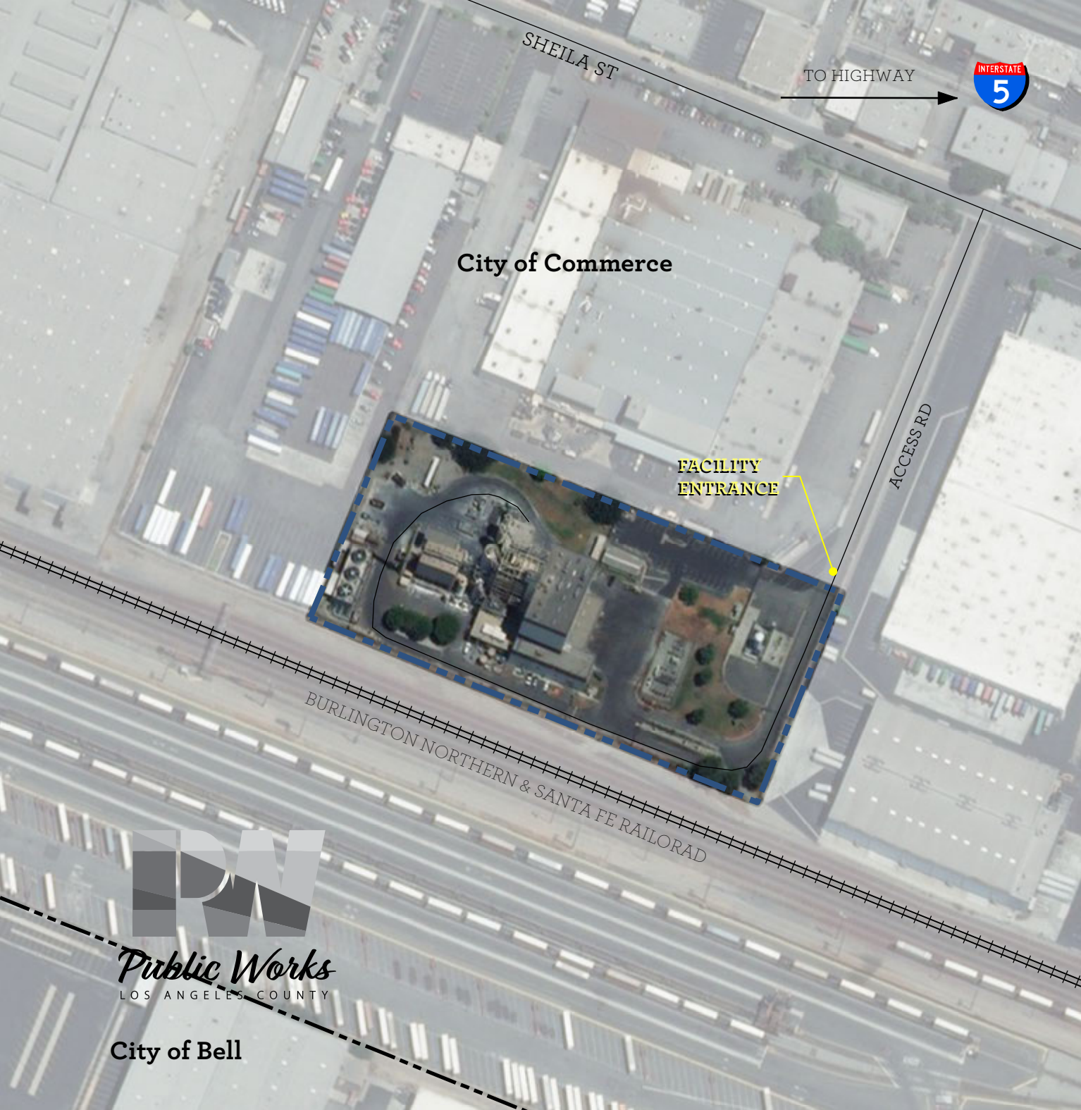
Figure 3-12: Commerce Refuse-to-Energy Facility (CREF) (closed as of 6/26/2018)
